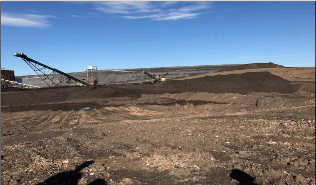
Figure 13-1: Rollover, Belt Conveyors, Stackers, and Stockpiles
